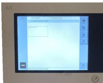
Figure 2 Laboratory Model: B&R Power Panel 500 – HMI display, placed on the front panel of the switchboard
